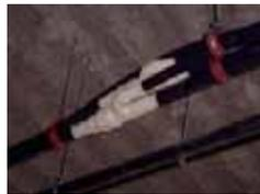
Support both sides of Y-joint and header.
