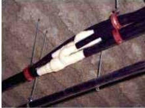
Support both sides of Y-joint & header.
