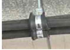
Additional piece of Insulation (prevent from insulation damage)
