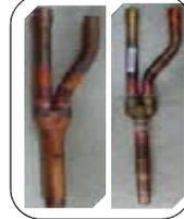
Incorrect installation of Y-joint & header joint cause poor oil and refrigerant distribution between IDUs. It may decrease the system's performance or cause compressor failure.
