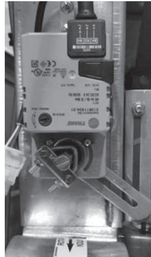
Figure 6. Actuator clamp position
