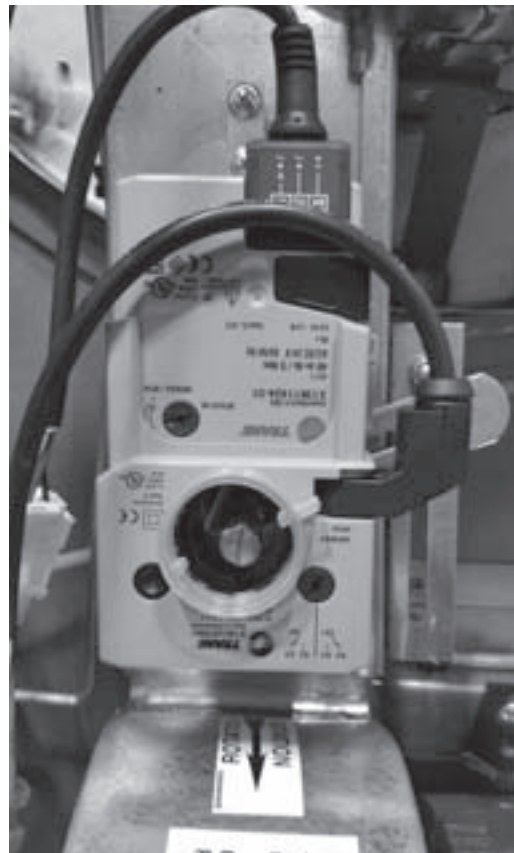
Figure 8. Auxiliary switch setting (full open)
