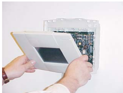
Figure 17: Display module installation
