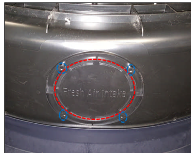
Figure 6 Circular Cassette External Knockout Locations
