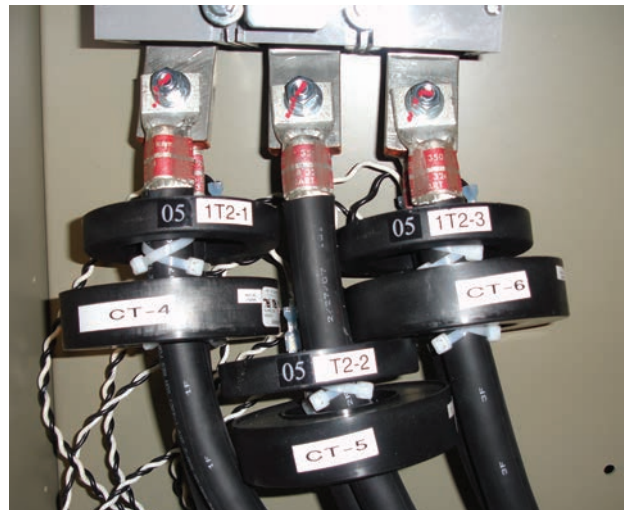
Figure 39. RTHD - Installation of CTs
