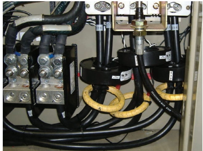
Figure 39. RTHD - Installation of CTs
