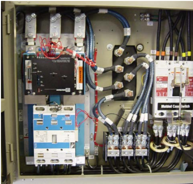
Figure 20. Location of Benshaw starter and additional components (highlighted)
