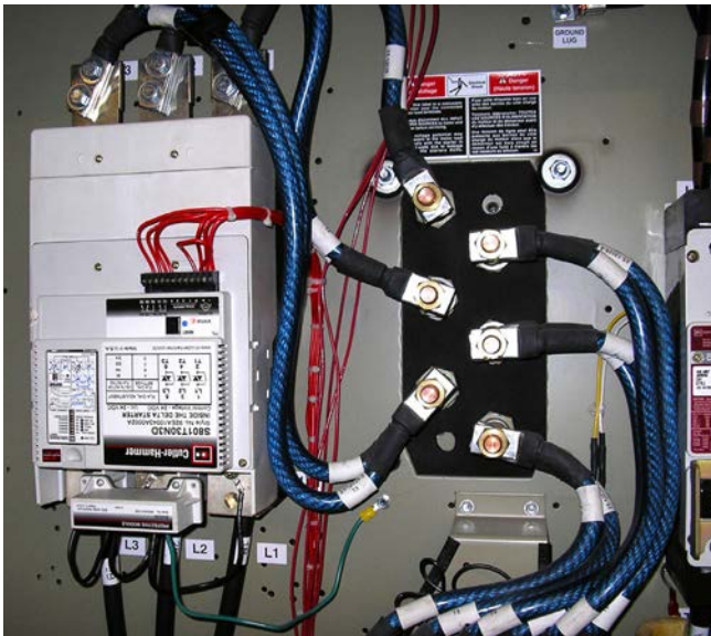
Figure 26. Location of Benshaw starter and additional components (highlighted) — RTHC
