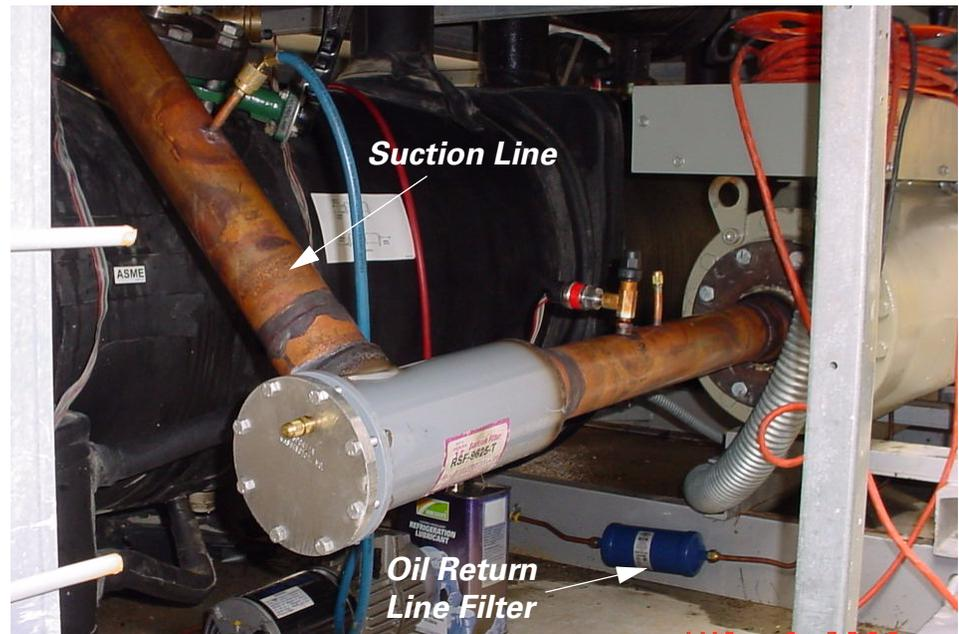
6. Install a small disposable filter core and sight glass on the oil return line from the bottom of the evaporator to the compressor. It is important that this filter is monitored to allow for oil return during the cleanup process. See Figure 2.
