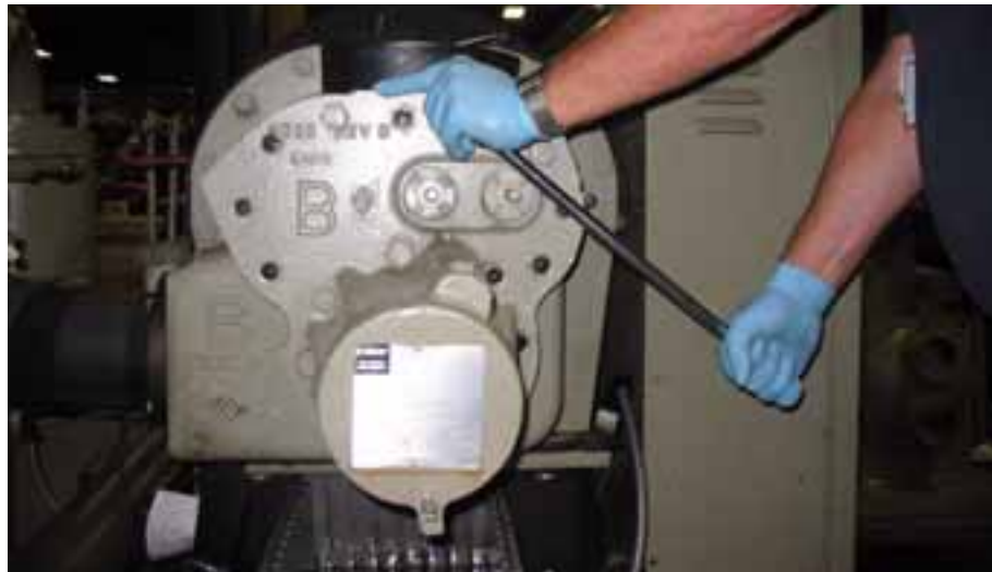
Figure 6. Removing Piston Housing Bolts
