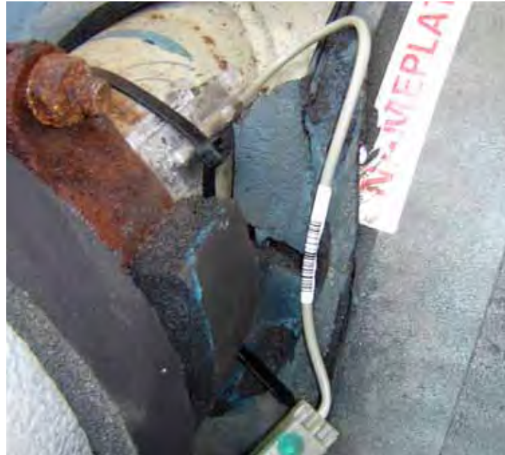
Figure 6. New evaporator entering water temperature sensor
