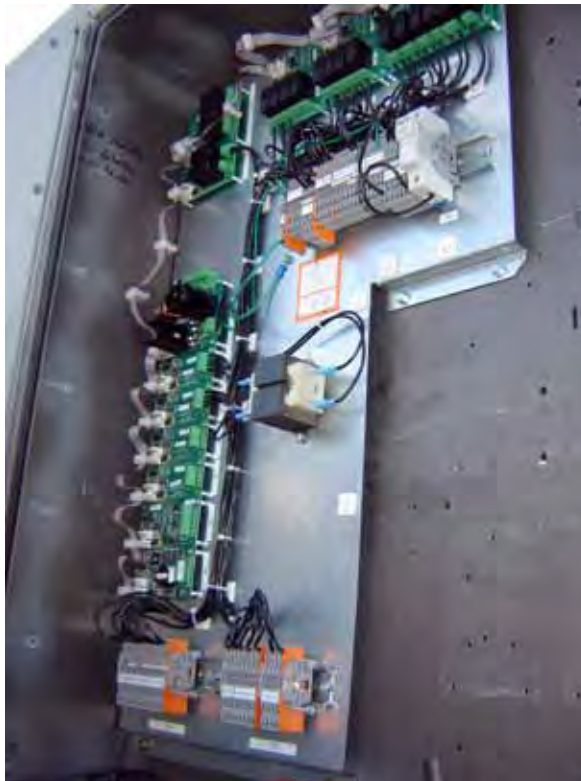
Figure 16. Panel section installed
