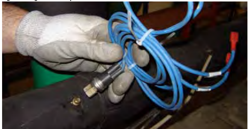
Figure 3. Original suction pressure switch location
