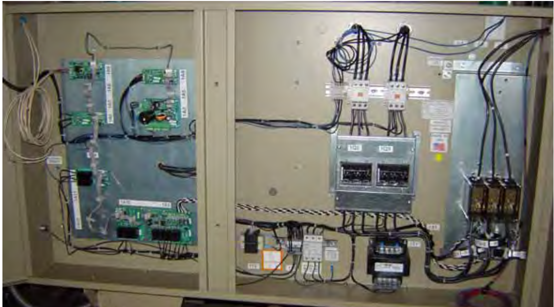
Figure 2. Water cooled panel after replacement
