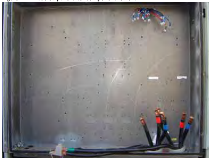
Figure 11. Air cooled panel after component removal
