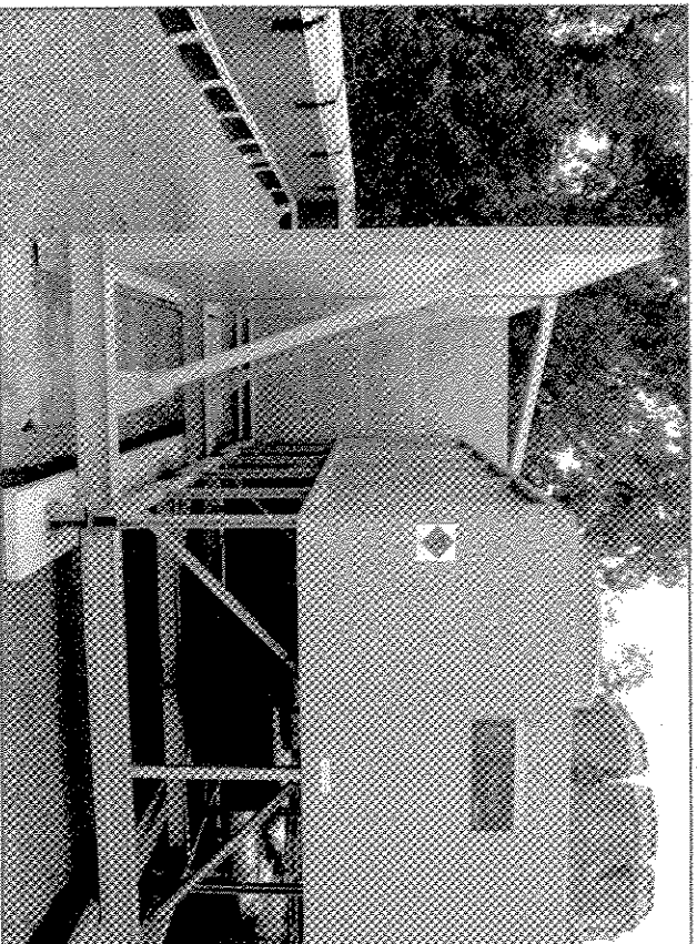
RTAA rooftop unit with HUSH GUARD™ barrier wall
