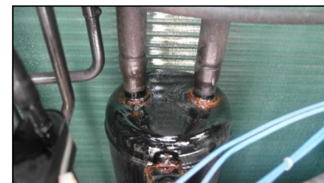
【Remove rust, and then Spray R-Pro on it】
