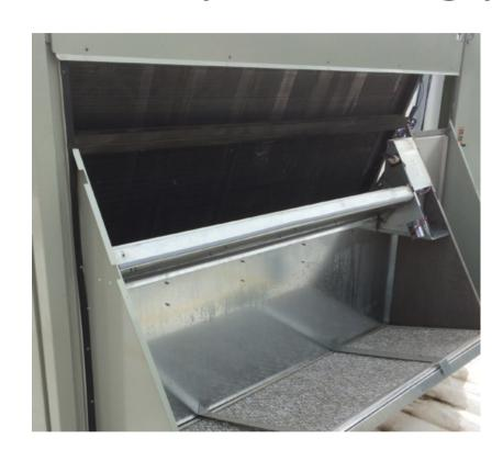
Unit end panel was removed for easier access of evaporator coil
