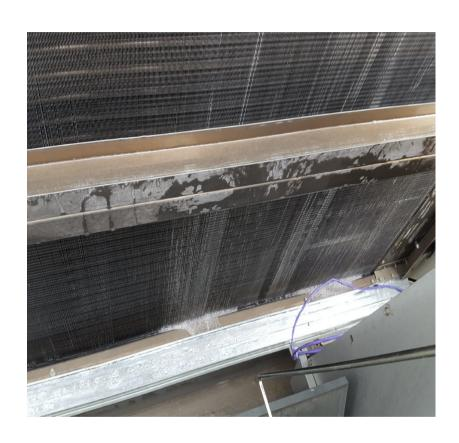
Technician rinsing off coil after cleaning
