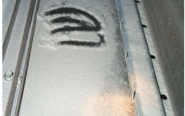
Figure 2. Drainpans are typically the first place that flakes accumulate. The amount of powder found can be noteworthy especially when no detectable breakdown of the fin surface is observed.
